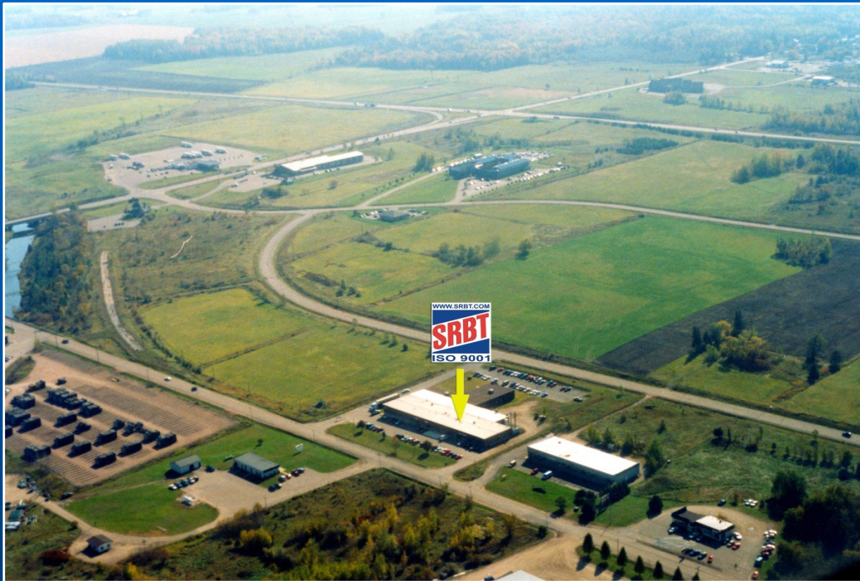
AERIAL PHOTOGRAPH OF THE FRONT OF SRBT'S FACILITY
